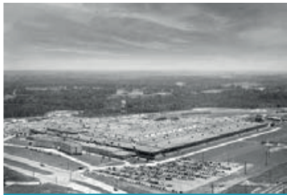
GM Assembly Plant in Doraville
