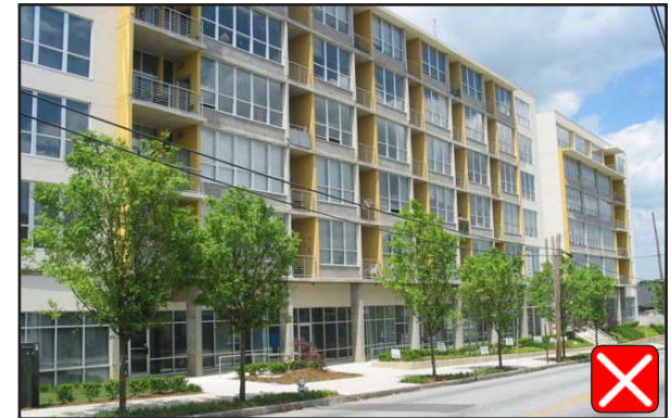
Multifamily residential buildings with a modern look ranked poorly
