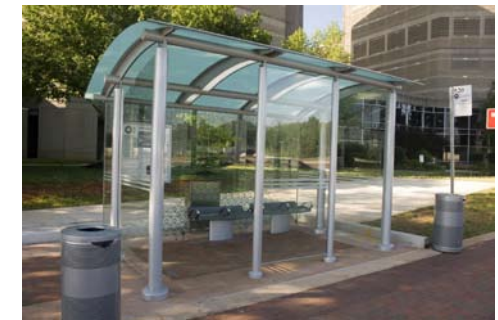
MARTA bus stop on Memorial Drive
